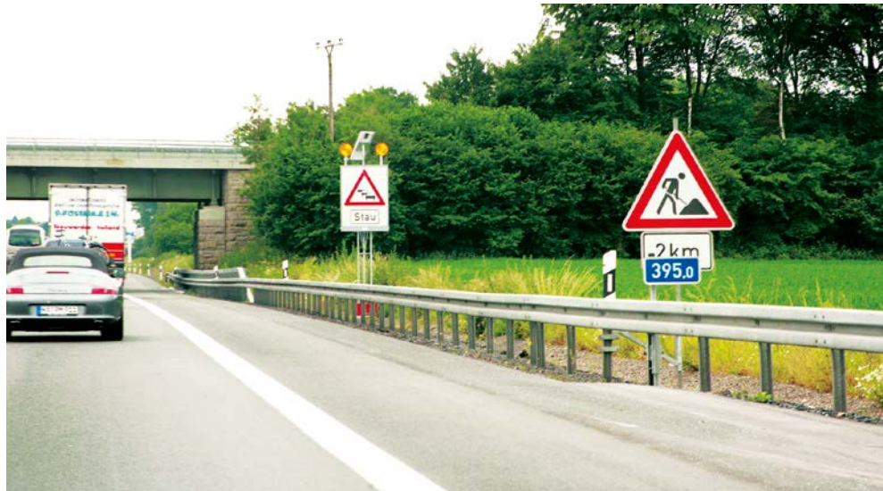
Safely (?) mounted traffic sign on a vehicle restraint system.
