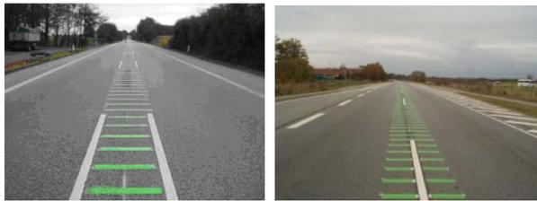
**Bild 2.22: Centre line marking, design A (li), design B (re) (HERRSTEDT, 2006)**
