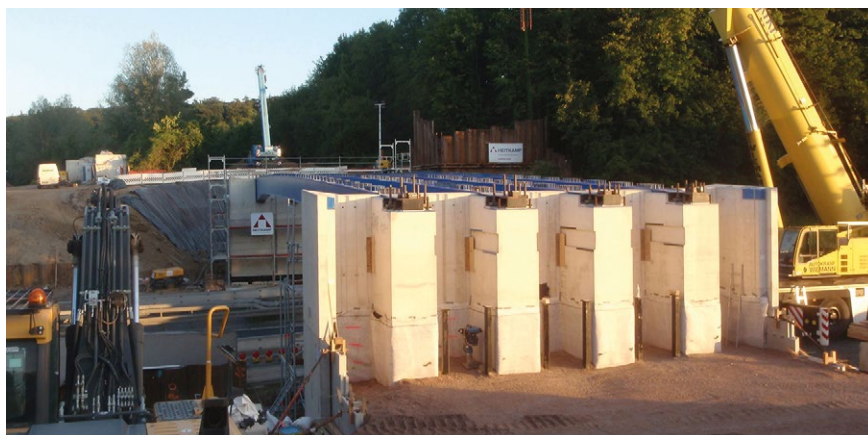
Overpass structure in modular design
