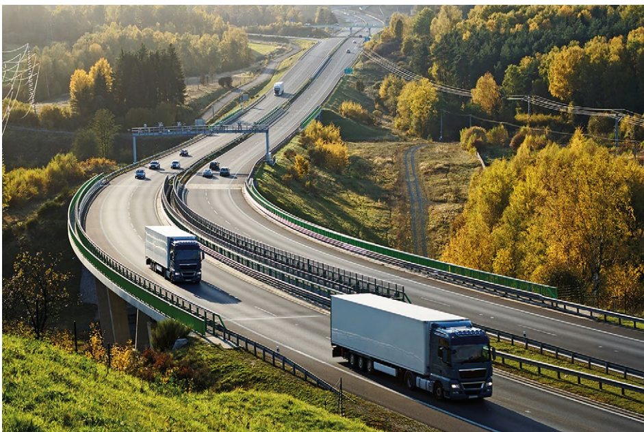
Asphalt motorway bridge with electronic toll point (© am/Fotolia)
