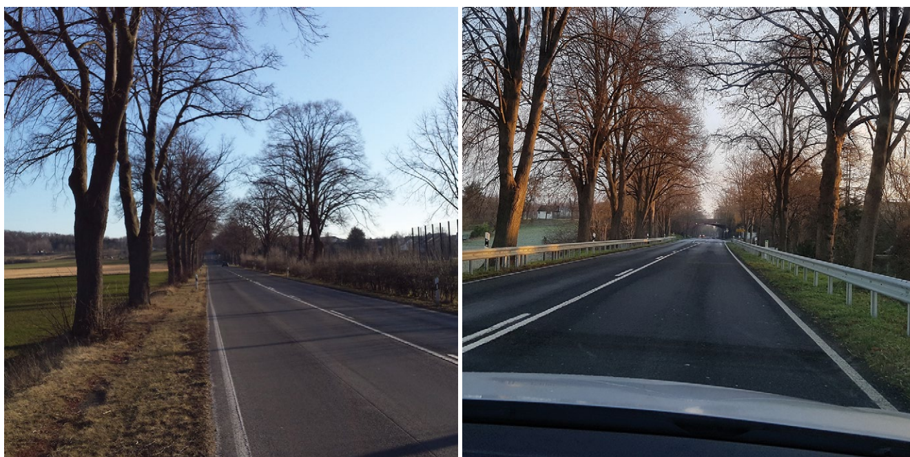
Rural road before (left) and after (right) being secured with safety barriers
