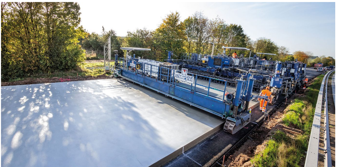
Installing a concrete pavement (picture: Schnorpfeil)
