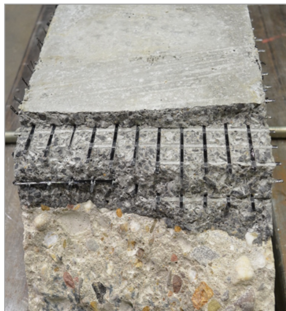
Figure 2: CRC layer after failure (cracking of carbon reinforcement).
