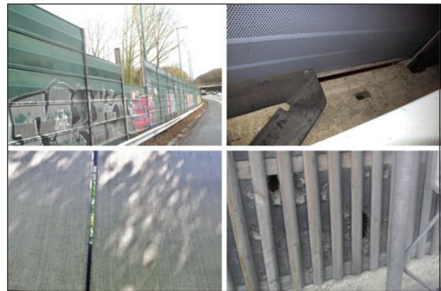
Fig. 4.1: Diverse defects at noise barriers; from top left to bottom right: absent aluminum element of noise barrier, leakage in the shape of a slit due to absent ground sealing, slit due to absent sealing between concrete elements of noise barrier, holes in insulating material of a wooden noise barrier due to mechanical impact (sources: BMVI; Walloon Road Administration, Belgium)
