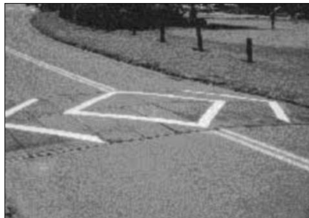
Figure 24: Speed hump in Athens
