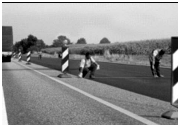
Figure 32: Construction site; source: DVR
