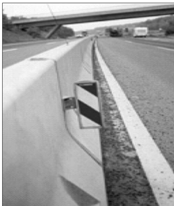
Figure 28: New Jersey elements on the M0 Budapest Ring Road; source: KTI
