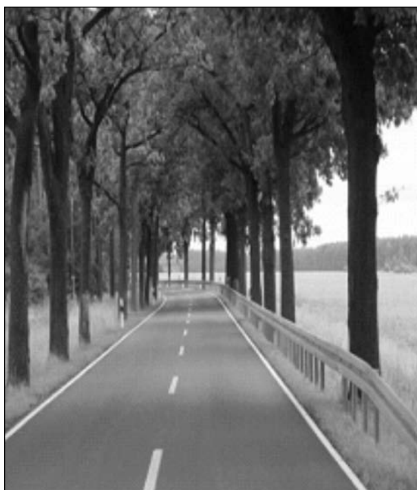
Figure 27: Guard rail; source: BAST
